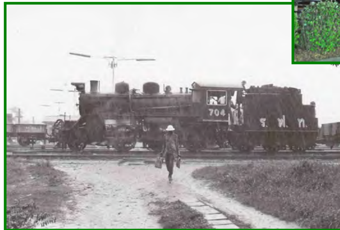
Switching in the Monsoon
