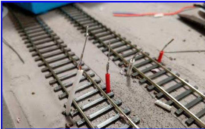
FIGURE 3—FEEDER 'TREES' PRIOR TO CONNECTION TO TRACK (USING CVT TIES AND GLUED RAIL)
